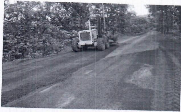
Photo # 4 - Haul road maintenance by Grader application AND Photo #5 Showing Trucks and Dumpers Covered With Tarpaulin
