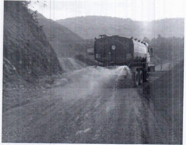
Photo #1C showing dust suppression by water sprinkling
