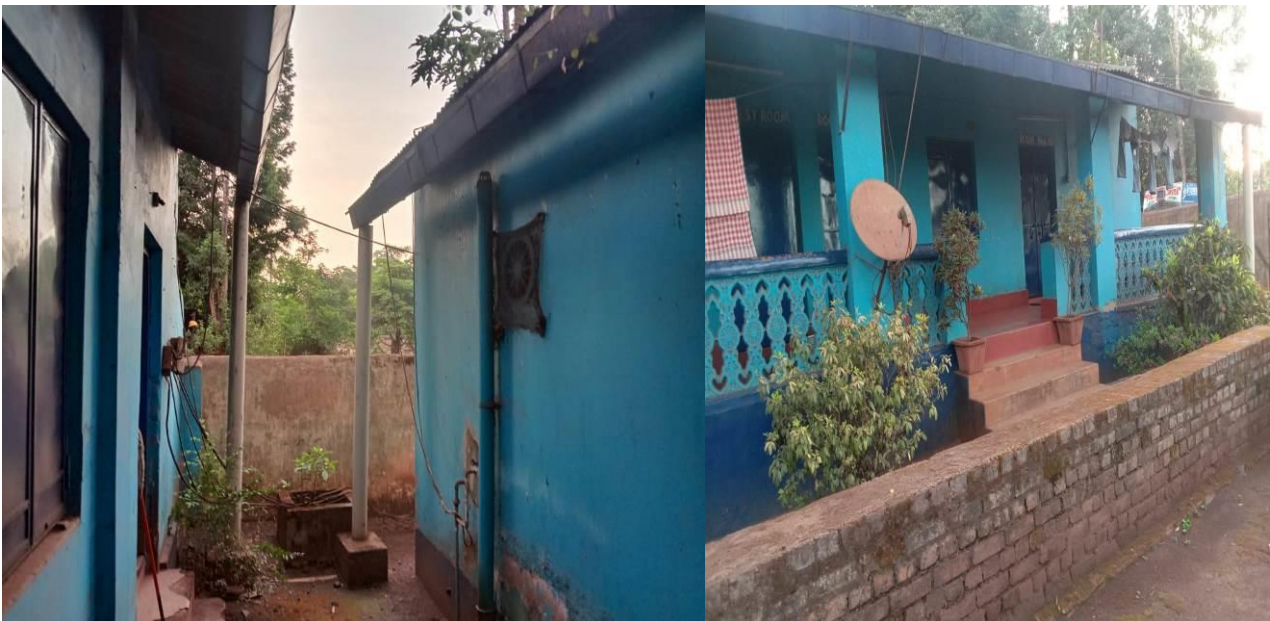
Photo # 3 - Showing rooftop rainwater harvesting measures at the camp area
