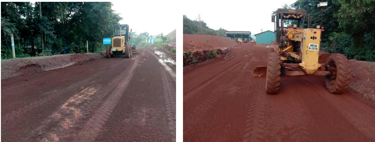
Photo # 4 - Haul road maintenance by Grader application
