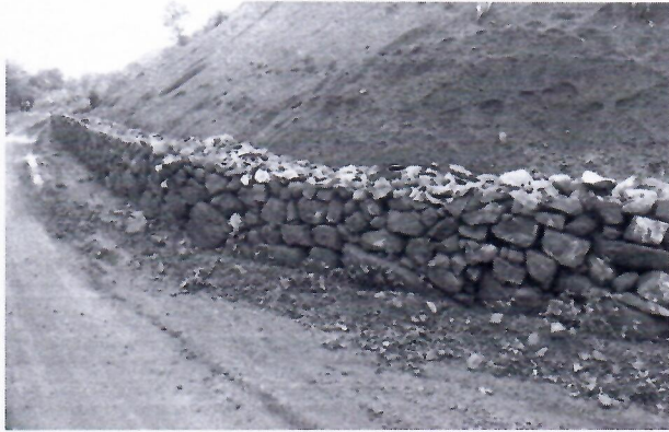
Photo #3 Showing Retaining wall & garland drain around OB Dumps
