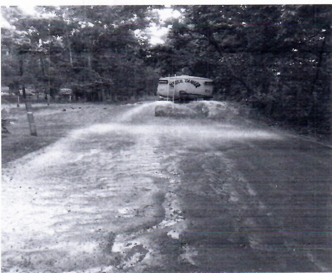
Photo #6 Showing 12 KL Water Tanker for Dust Suppression On the Haul Road
