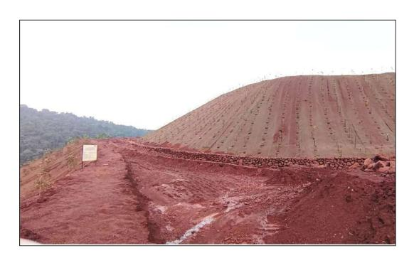
Photo #3 Showing settling cum harvesting pits along with check dam & check weir
