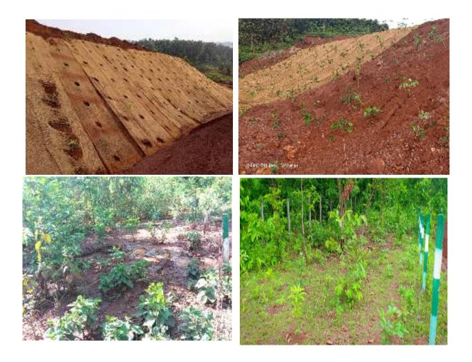
Photo #1B showing Retaining wall garland drain around OB Dumps & coir mat application for dump stabilization in the back filled areas
