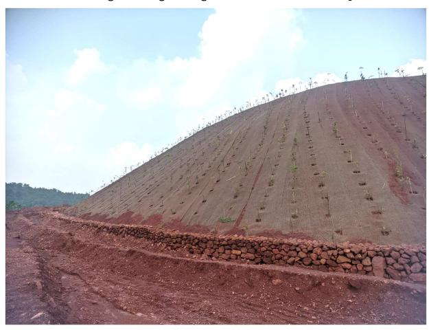
Photo #2 Showing Retaining wall & garland drain around OB Dumps
