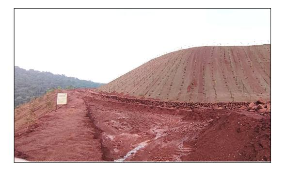
Photo #3 Showing settling cum harvesting pits along with check dam & check weir
