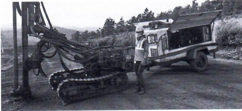
Photo #2 Showing Drilling Machine with Water Injecting System
