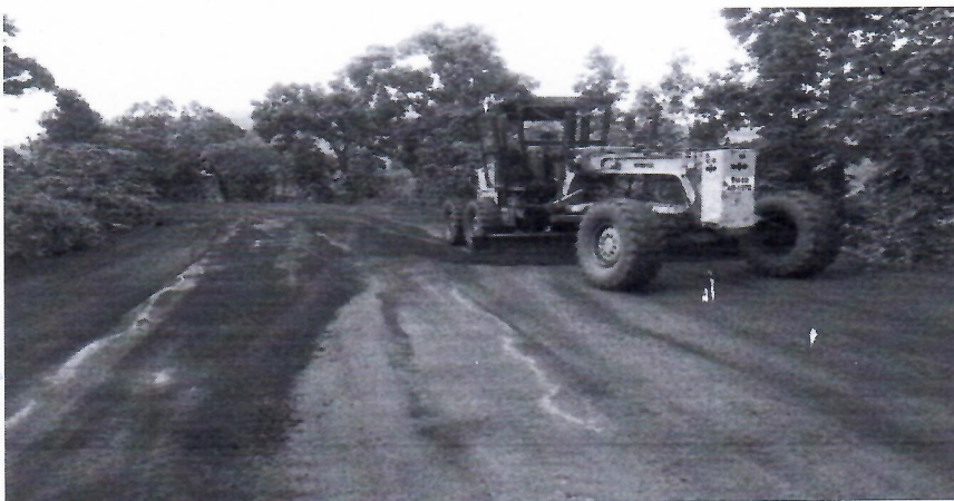
Photo #4 Haul road maintenance by Grader application
