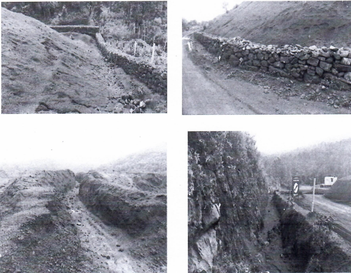
Photo #1B showing Retaining wall & garland drain around OB Dumps
