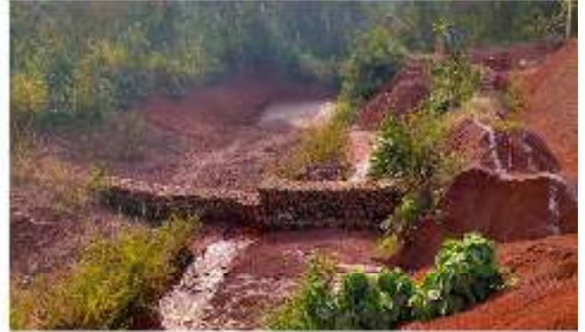
Photo # 6 showing Check Dam
