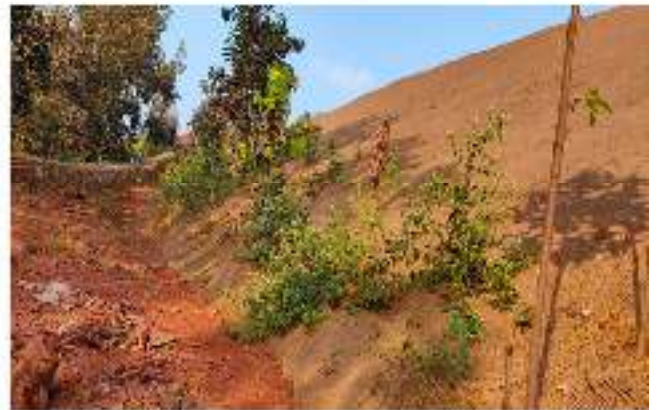
Photo # 7 showing Top Soil Stack inside the ML area with waste dump cover matting provisions & retaining wall at toe of the dump
