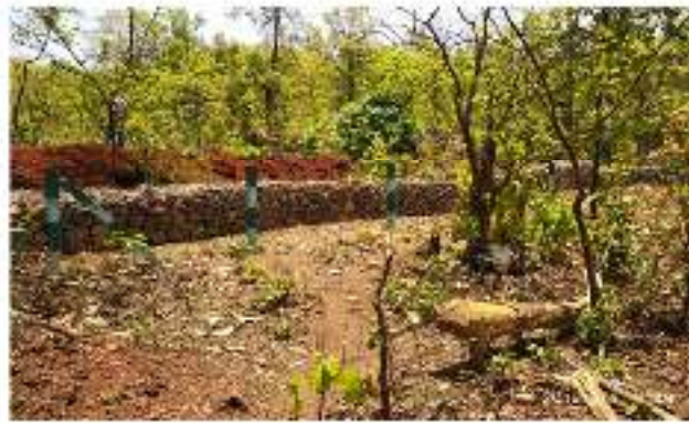
Photo # 1B showing Retaining Wall all along the Nala Safety Zone & strategic locations
