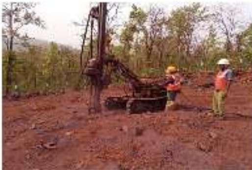
Photo # 2A Showing Drilling Machine with Water Injecting System
