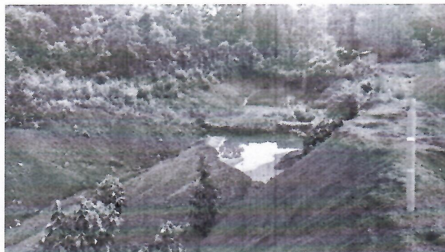
Photo # 3 & 6 - Showing settling tanks with check weir & check dams at strategic locations
