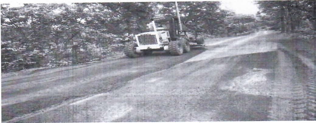
Photo #4 Haul road maintenance by Grader application
